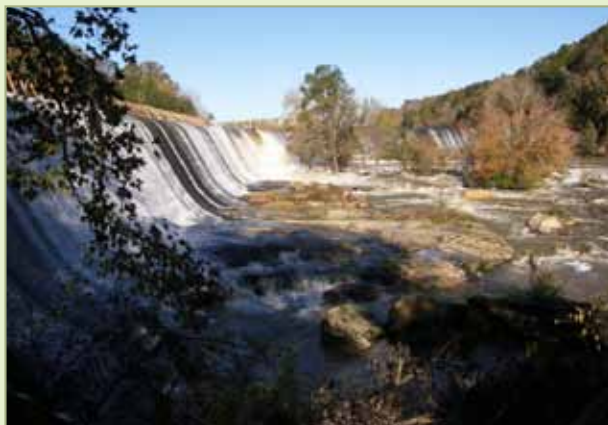
Headworks Dam in Great Falls Bill Stokes
