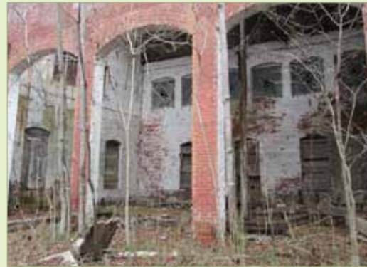
Nitrolee Building Barry Beasley
